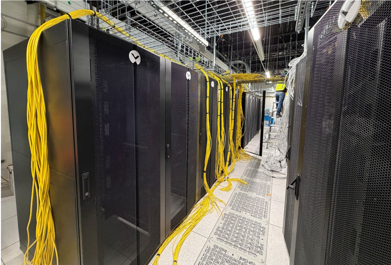
Data Centre, Final termination of structured cabling, March 12, 2026
