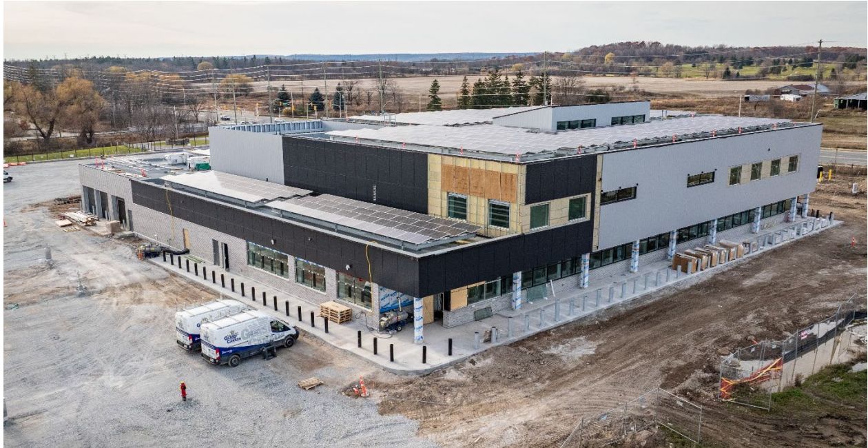
South East Elevation, Exterior metal siding nearing completion, sidewalks in progress – Nov 26, 2025
