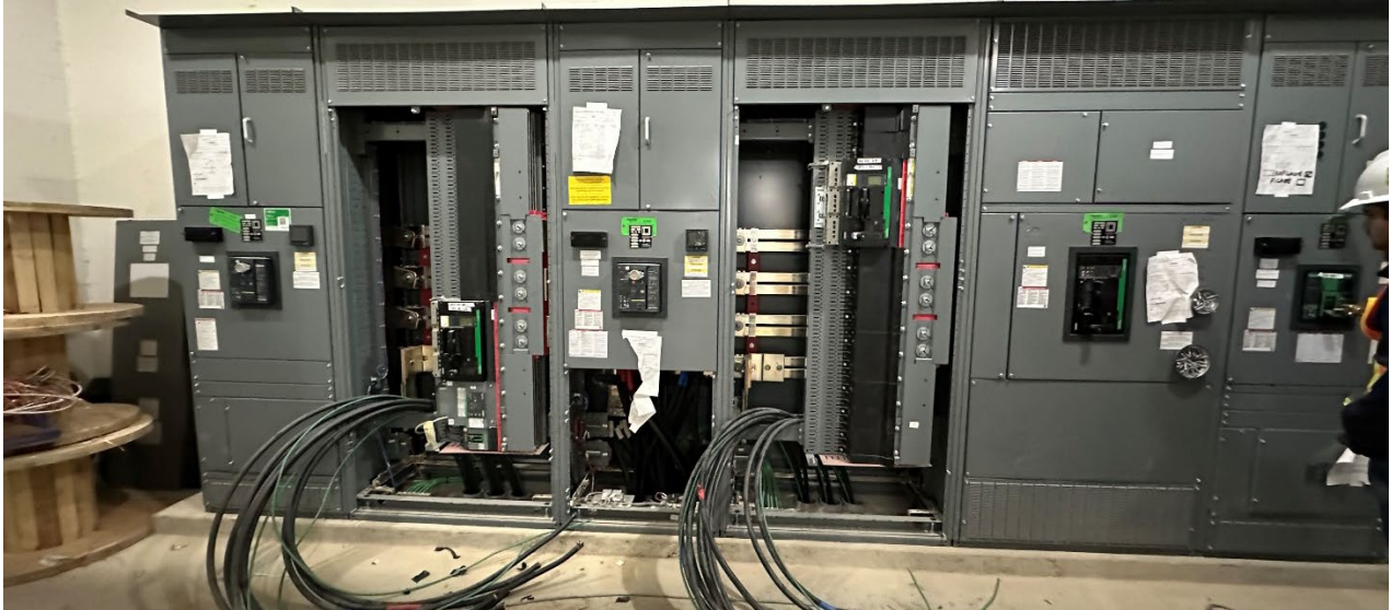
Electrical Room, installation of switch gear electrical feeders, Nov 27 2025
