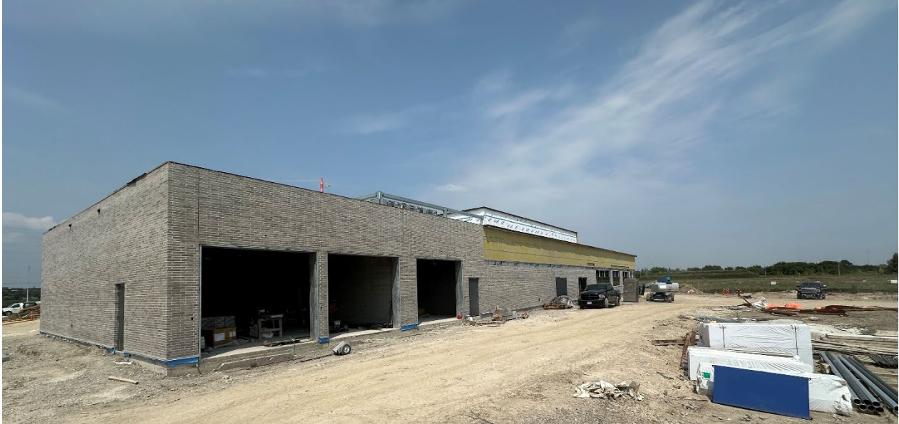
South West Elevation, brick veneer masonry installed – August 7, 2025
