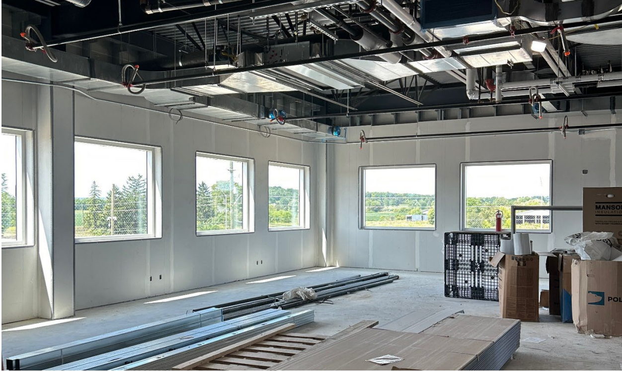
2nd floor, Drywall installation – Aug 21, 2025
