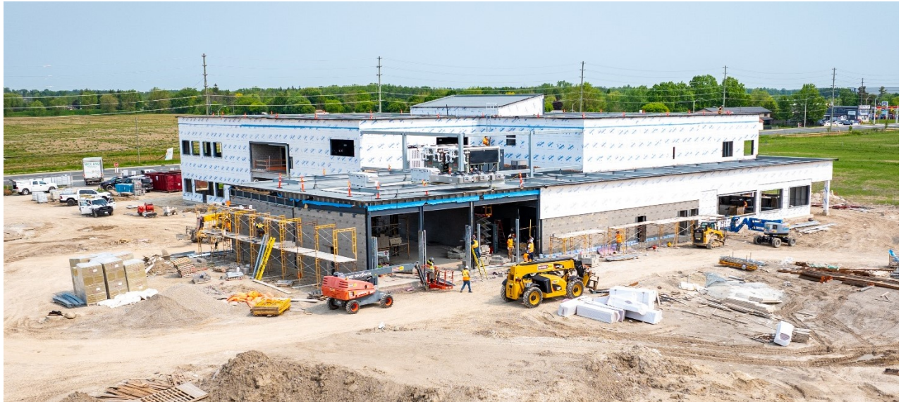
South West Elevation, overhead door framing in progress & exterior wall preparation for installation of masonry and metal panel finishes – June 3, 2025
