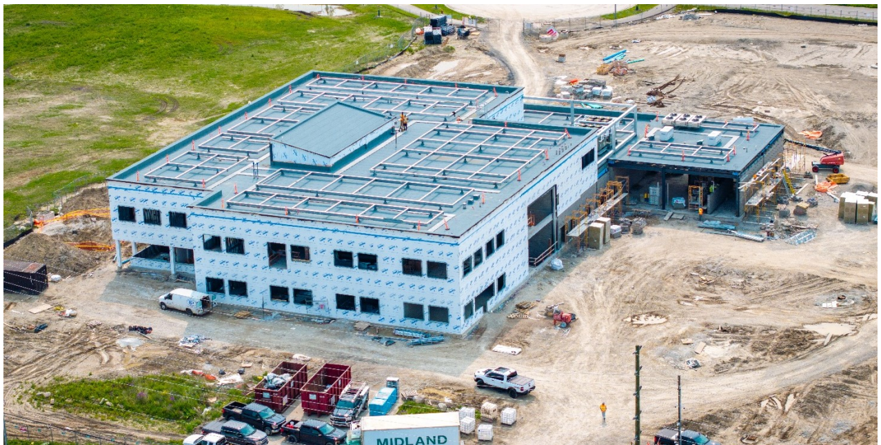
North West Aerial, roofing complete with solar panel structural supports installed & roof top mechanical equipment in place – June 3, 2025
