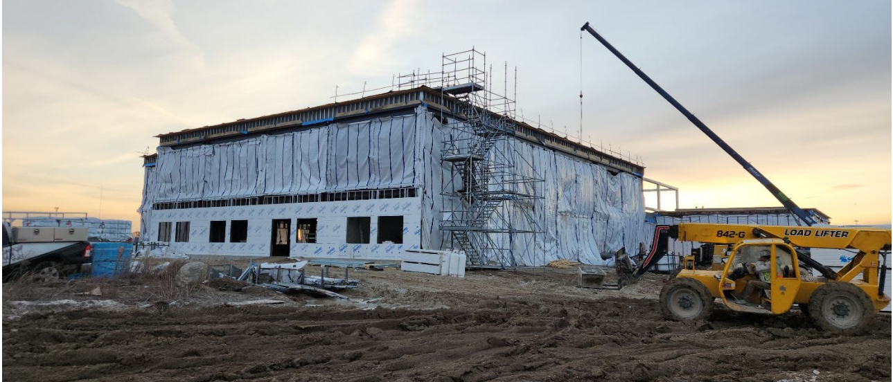
North Elevation, exterior wall stud framing and sheathing in progress – Mar 12, 2025
