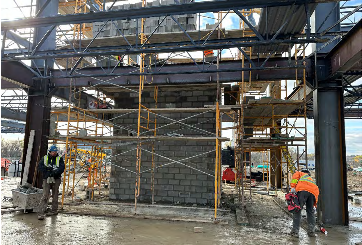
Main floor, Installation of masonry block for elevator shaft – Nov 28, 2024
