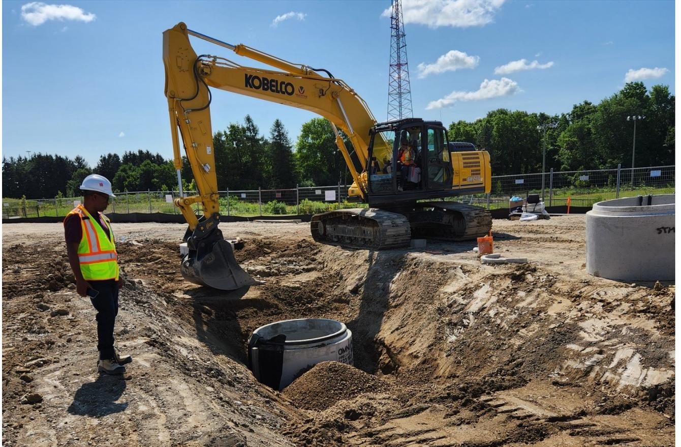
Installation of storm water catch basin – Aug 28, 2024
